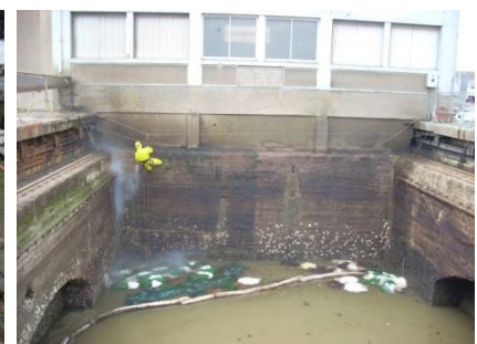
Photo 24 High pressure washing in port basin by a rope work specialist (source Cedre)
