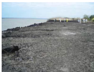
Photo 26 River banks just after cutting of common reed and sediment surface scraping (source Cedre)
