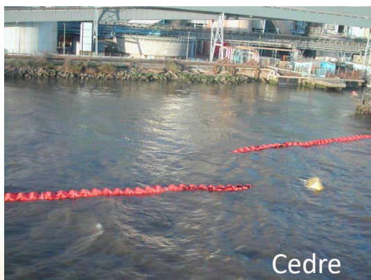
Water intake of the power station
